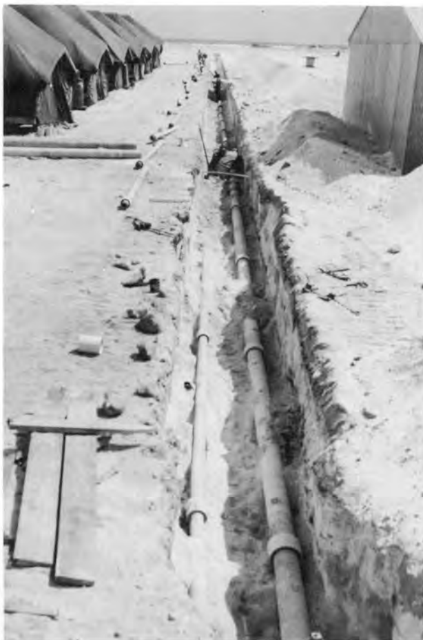
Figure 4-20. Fresh and Salt Water Pipe - Being Installed
